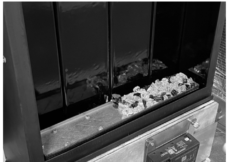
Burner Glass Media – Partially Installed
