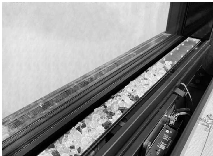
Burner Glass Media – Partially Installed
