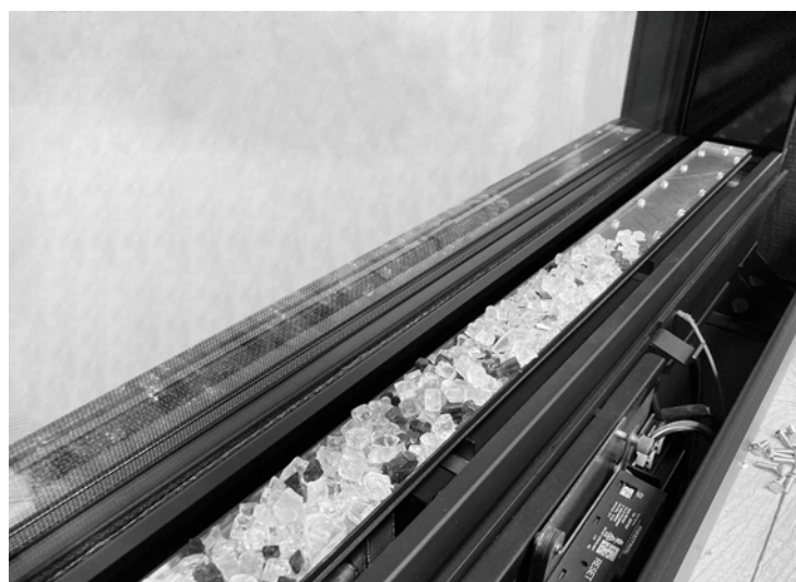
Burner Glass Media – Partially Installed
