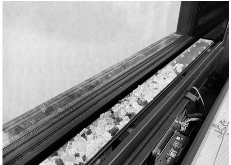
Burner Glass Media – Partially Installed
