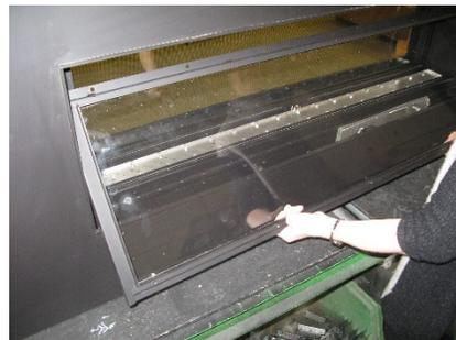
2. Lift the glass frame assembly up so that the bottom of the glass frame assembly clears the bottom of the fireplace opening.
