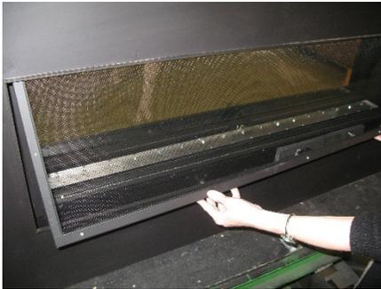
3. The fireplace screen is held in place by 3 self-tensioning latches along its top edge (4 latches on the SEVENTY2). Release these latches to remove the screen.
