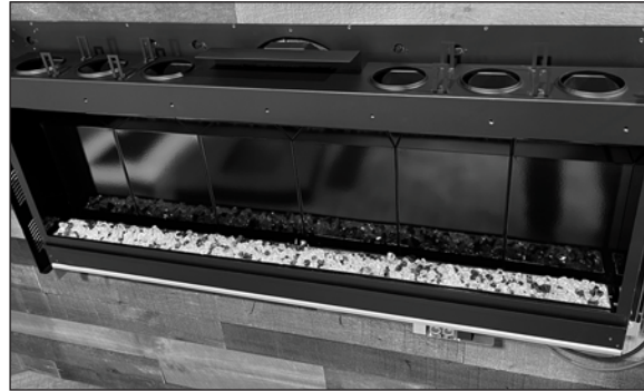
Burner Glass Media fully installed
