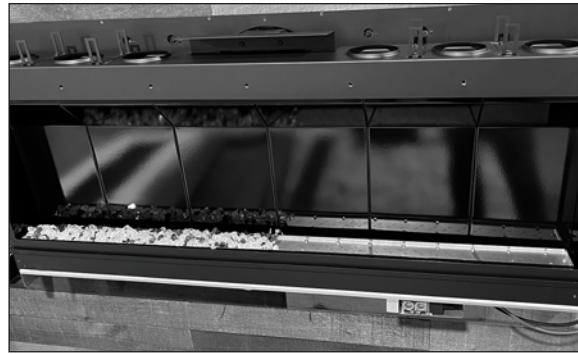
Burner Glass Media partially installed
