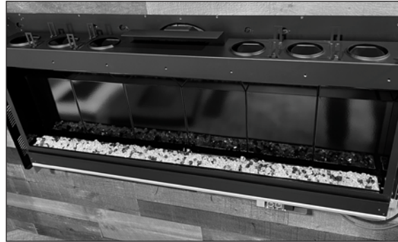
Burner Glass Media fully installed
