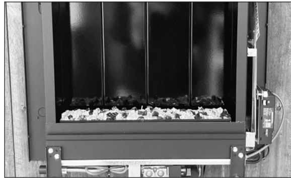
Burner Glass Media fully installed
