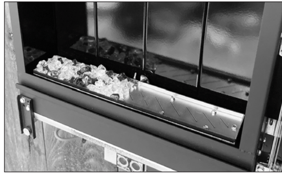
Burner Glass Media partially installed
