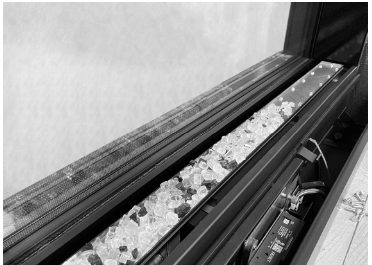
Burner Glass Media – Partially Installed
