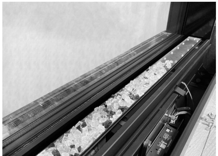
Burner Glass Media – Partially Installed
