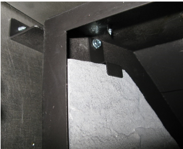
3. At the top of the left liner panel, install the top retaining clip, part # 12367 as shown.
