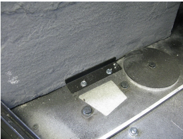
2. At the base of the left liner panel, install the base retaining bracket, part # 12366, as shown.
